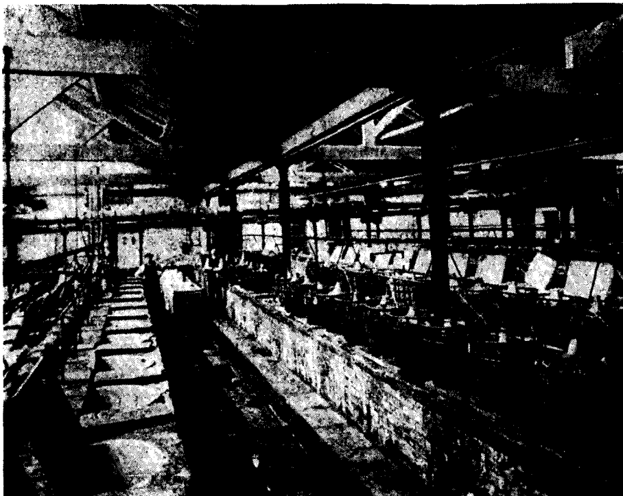
FIG. 117. General view of nitrators for the production of picric acid [8].
